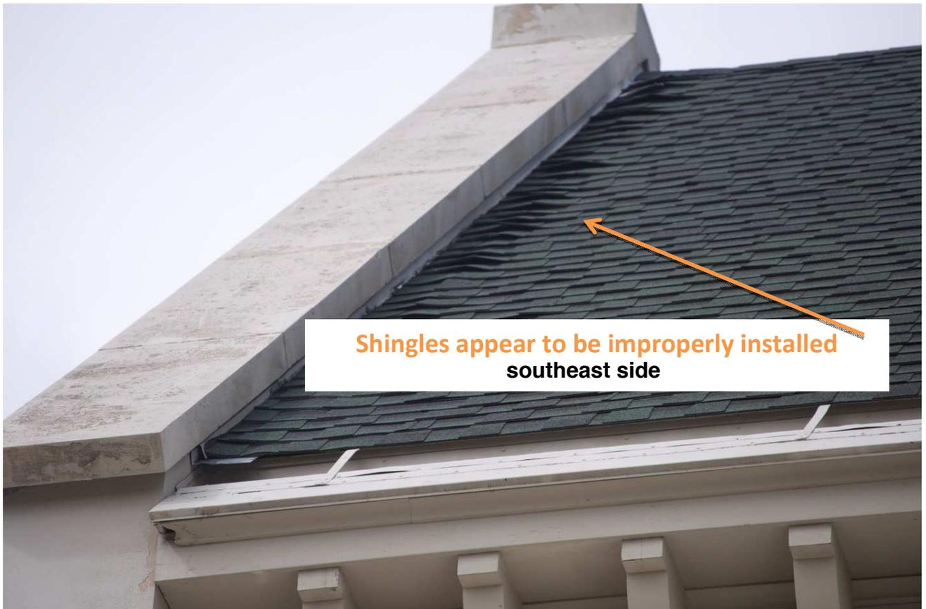
**Shingles appear to be improperly installed
