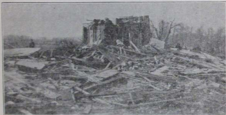
RUINS OF FLOYD BASCOM'S HOME ON THE F. J. CONKLIN FARM AFTER THE CYCLONE OF MARCH 28, 1920
