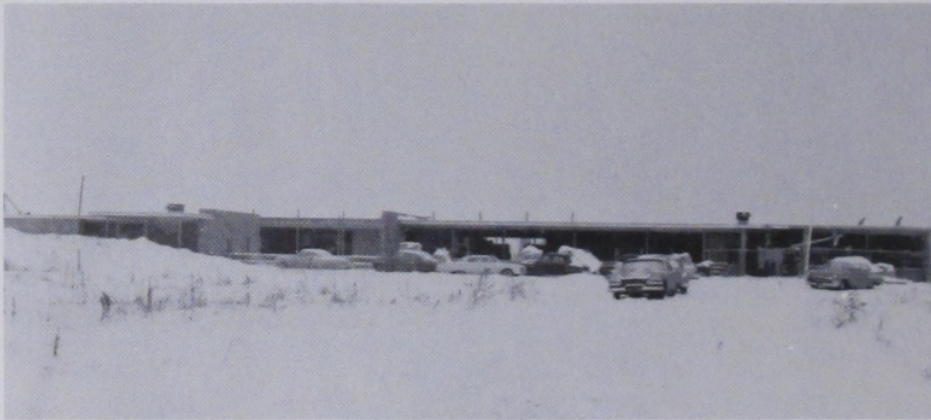
Construction of the new high school
