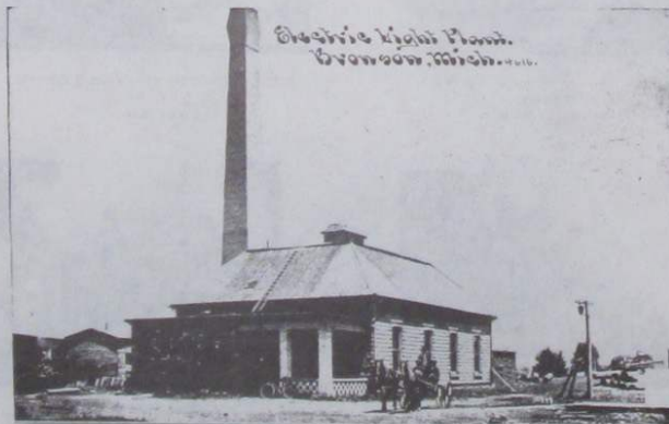
ELECTRIC LIGHT PLANT, BRONSON, MICH.
