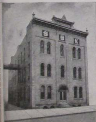
KITCHEL'S LINIMENT LABORATORY AND NEWSPAPER OFFICE.
