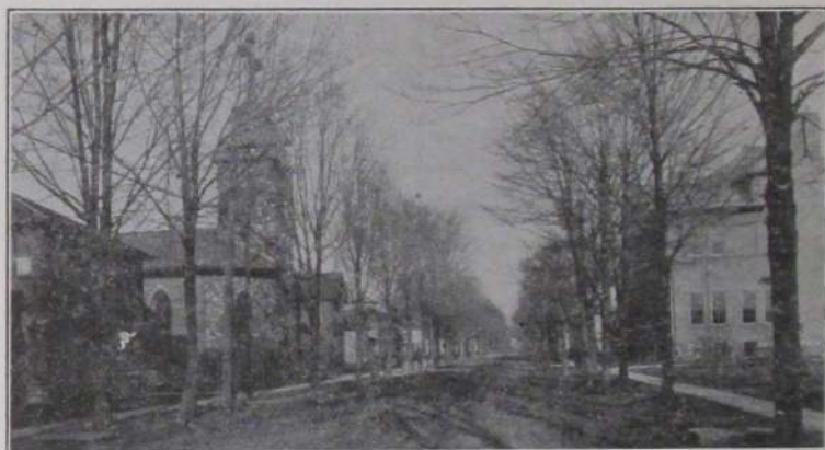
VIEW ON HARRISON STREET, SHOWING ST. CHARLES CHURCH'S FOUR BUILDINGS
