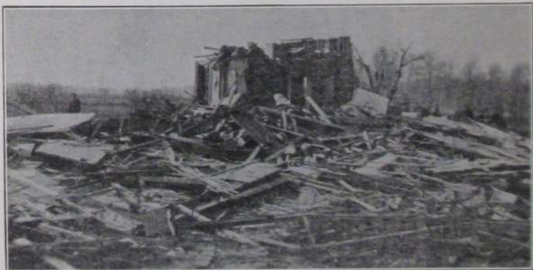
HOME OF FLOYD BASCOM ON THE F. J. CONKLIN FARM AFTER THE CYCLONE OF MARCH 28, 1920
