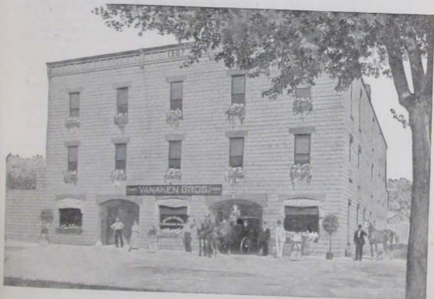
THE VANAKEN BLOCK, DESTROYED BY FIRE JULY 15, 1920
