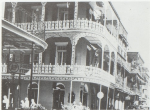
Lace balconies were to be seen everywhere.
