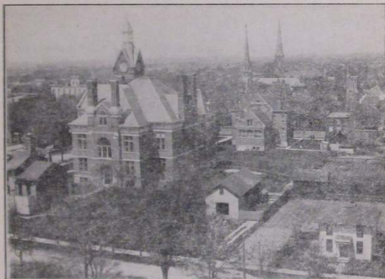
Birdseye View from the Tower of the Lincoln School Building
