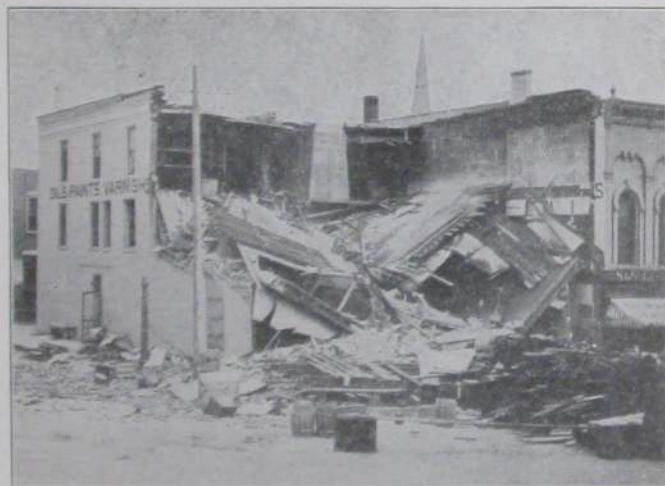
THE E. R. CLARKE & CO. BUILDING AFTER THE COLLAPSE OF OCTOBER 6, 1913
