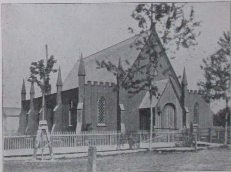
OLD EPISCOPAL CHURCH, ERECTED IN 1862
