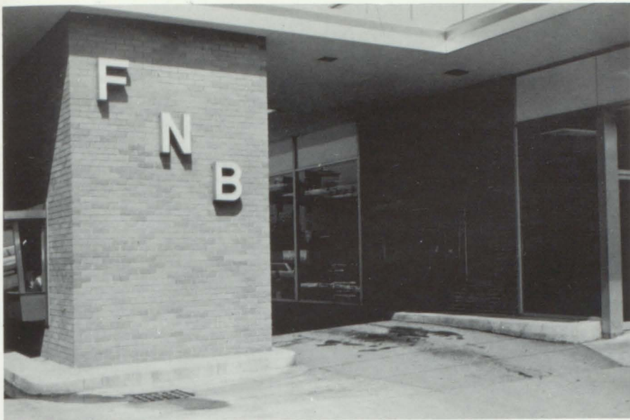
The bank provides "drive-in" windows for those on the go.
