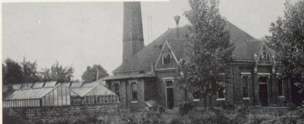
Waterworks Park in Quincy just north of the railroad.
