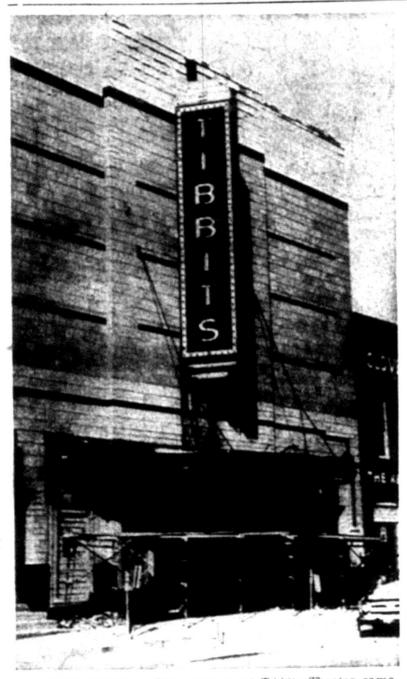
coming down—The marquee at Tibbits Theater came down Thursday and today workmen were dismantling the large electric sign. The tile facing on the front of the theater is slated to be removed next in a program designed to restore the exterior to its "opera house" days. Whether the bust of Shakespeare is still in a niche high on the facade behind the tile will be discovered soon. (Daily Reporter photo)
