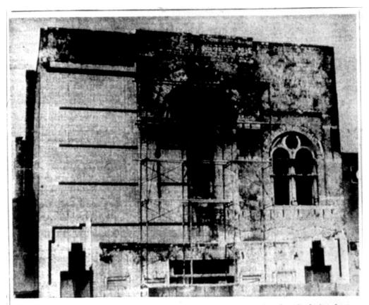
FACE CHANGING — Workers are making progress in removing the tile facing from Tibblits theater, revealing the old brick and stone facade that marked the building back in its "opera house" days. Plans call for eventual restoration of the front to its original appearance. Above photo shows progress to date. (Daily Reporter photo)
