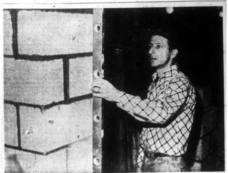
MANY HANDS are helping with the rejuvenation of historic Tibbits theater. Karl Staley, local mason and carpenter, places a level on a wall of the concrete block furnace room being constructed in the basement. Russell Belt and Stanley Cuthbert have also been helping with this portion of the work—all three donating their time and skill in the current campaign to restore the theater building for community use. (Daily Reporter photo)
