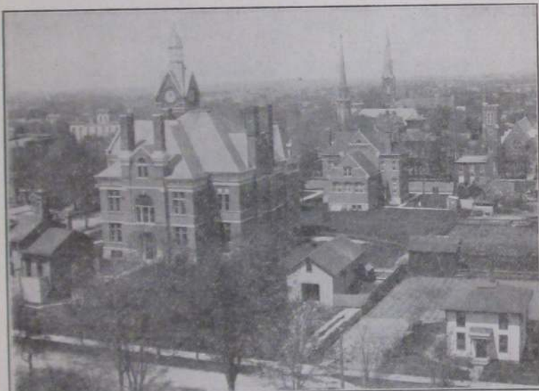
VIEW FROM THE TOWER OF THE LINCOLN SCHOOL BUILDING
