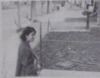
YARD UNDER CONSTRUCTION
