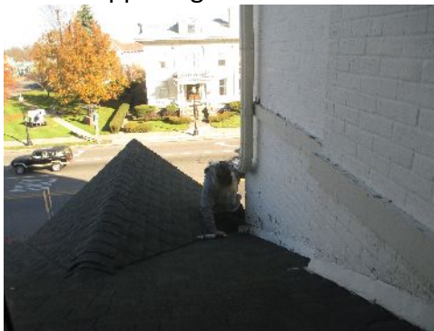
Is this Santa checking the roof?
